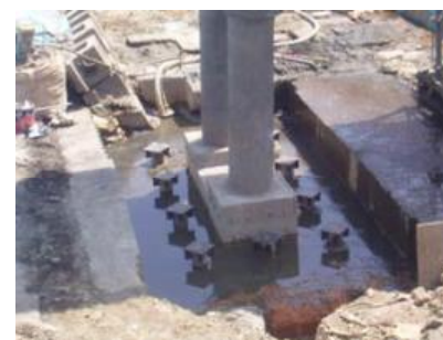
(頭部支圧板溶接完了)
