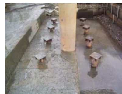
(頭部支圧板溶接完了)
