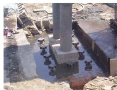
(頭部支圧板溶接完了)
